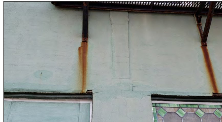
FRONT FAÇADE CONDITION
