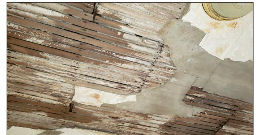
TYPICAL CEILING WATER DAMAGE
