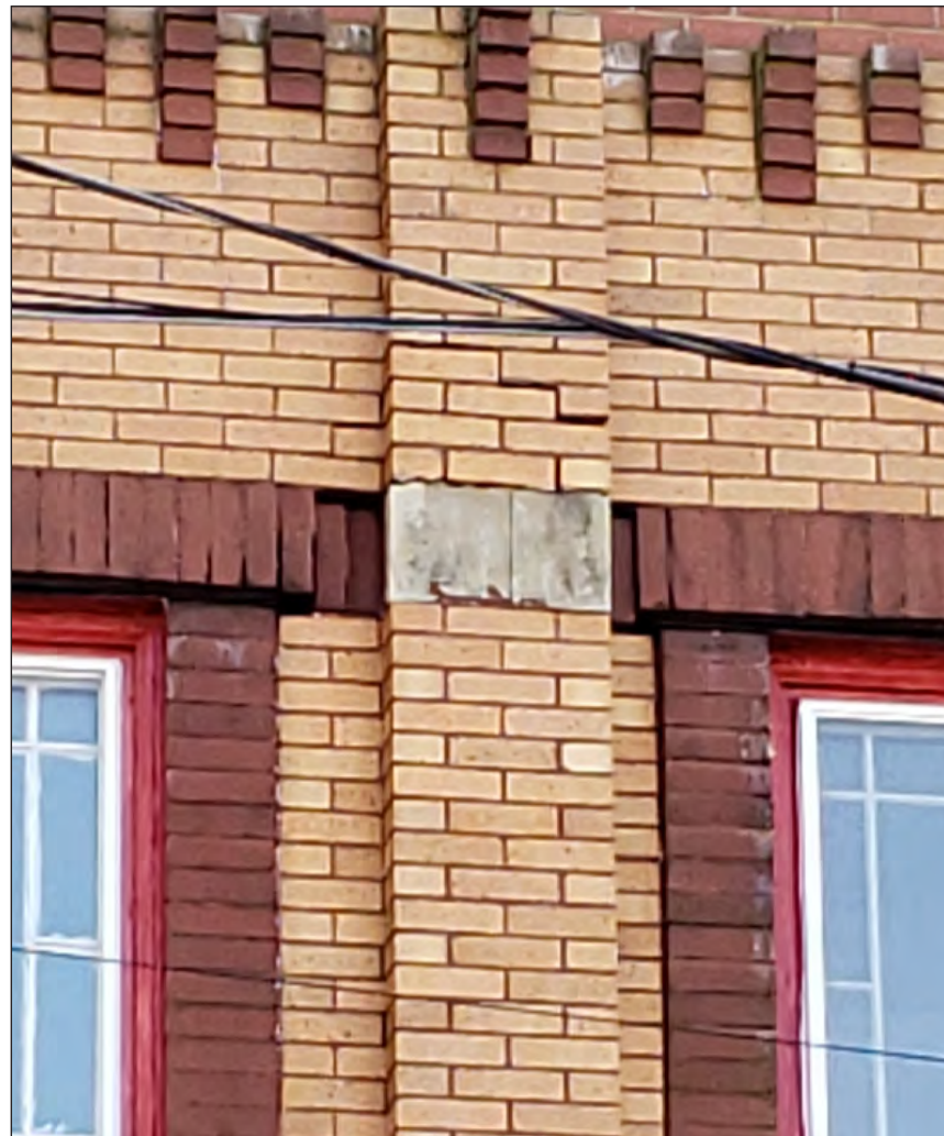
FRONT FAÇADE CONDITION
