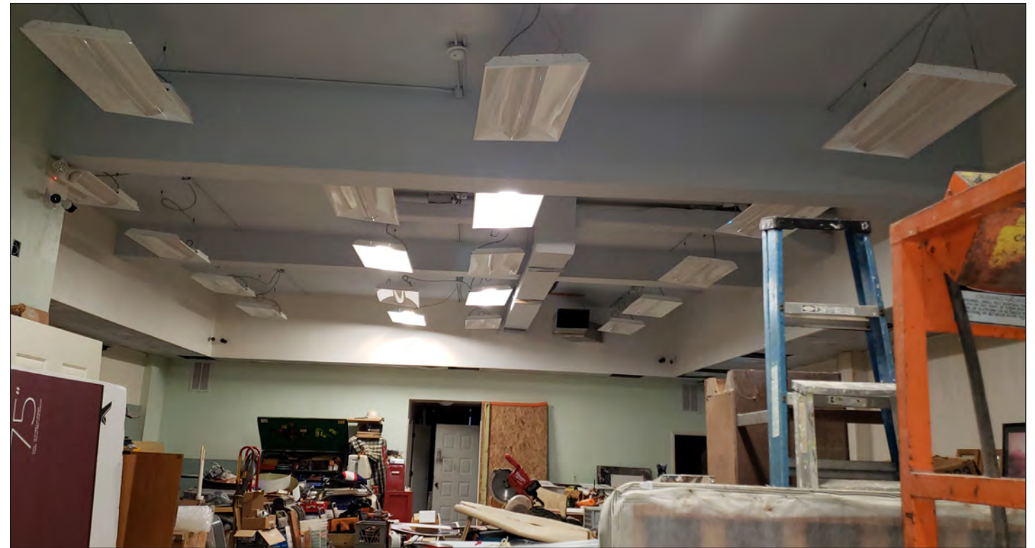
TYPICAL INTERIOR CONDITION
