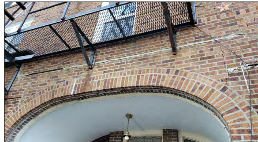
FRONT FAÇADE CONDITION
