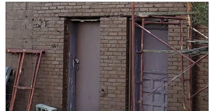
TYPICAL LINTEL/MASONRY CONDITION
