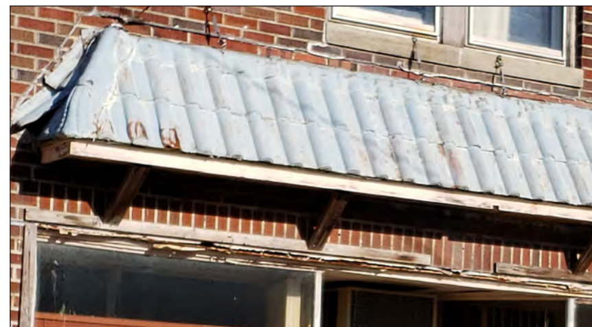
TYPICAL LINTEL CONDITION
