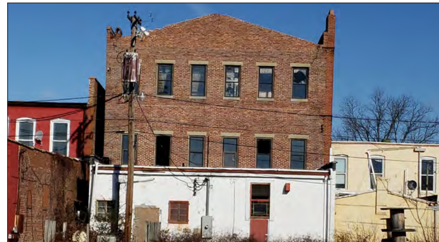
REAR FAÇADE CONDITION
