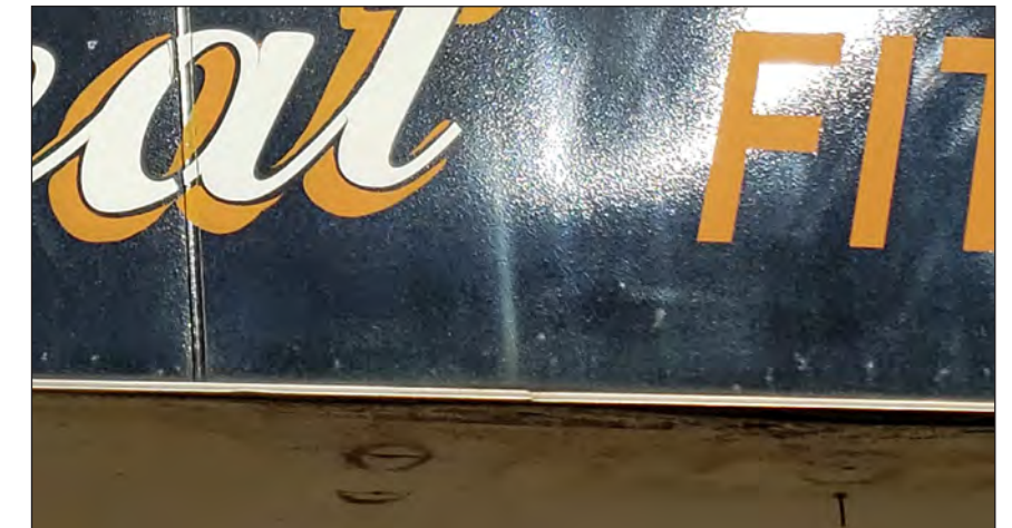
386 W. MAIN STREET STORE FRONT CONDITION
