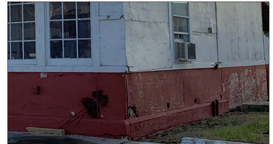
EAST FAÇADE CONDITION
