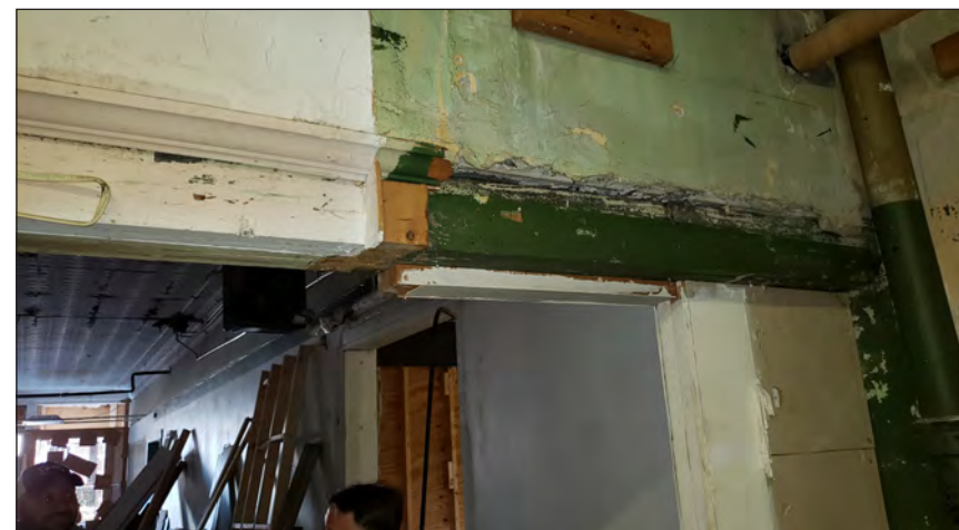
LINTEL CORROSION
