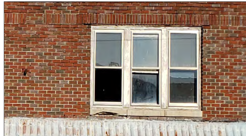
TYPICAL WINDOW CONDITION
