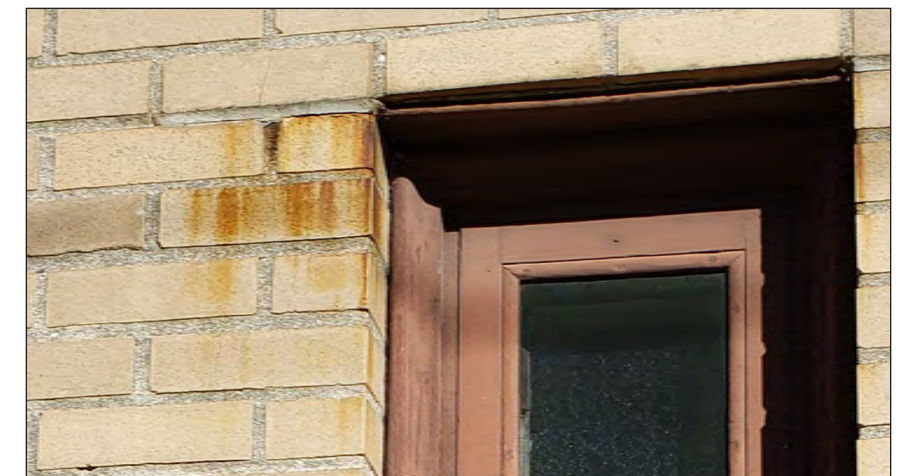
FRONT FAÇADE LINTEL CORROSION
