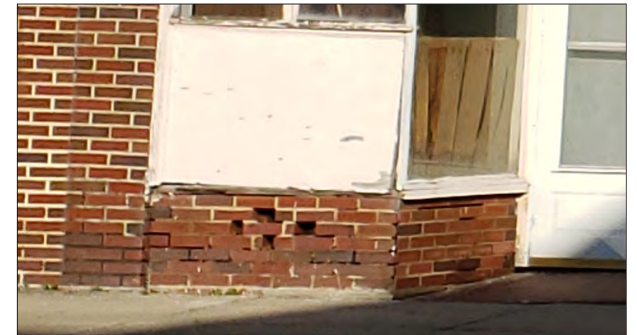
DISPLACED/MISSING MASONRY UNITS
