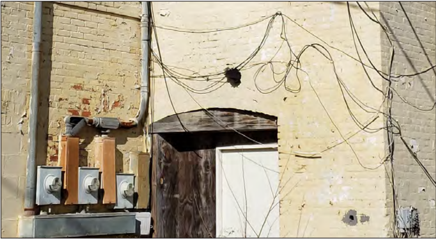
REAR FAÇADE CONDITION
