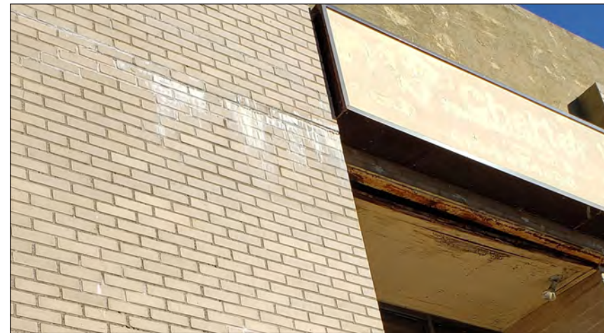
EFFLORESCENCE AND SHELF DAMAGE
