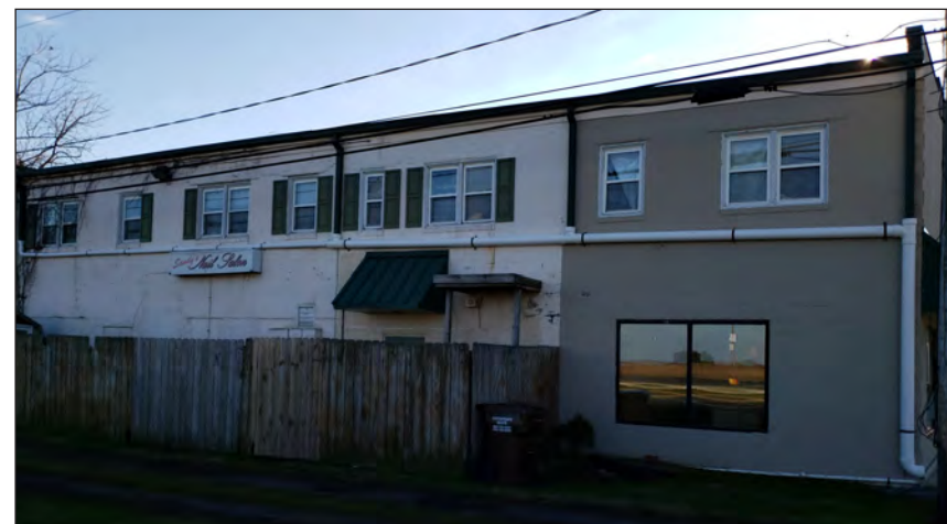
REAR FAÇADE CONDITIONS
