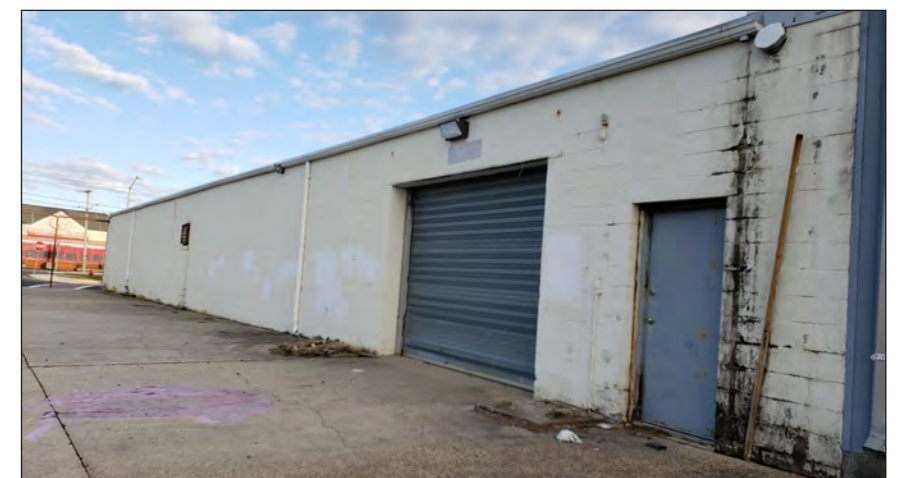
WEST FAÇADE CONDITION
