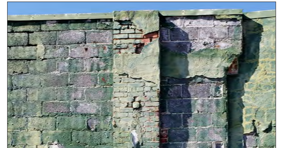
TYPICAL CMU WALL CONDITION
