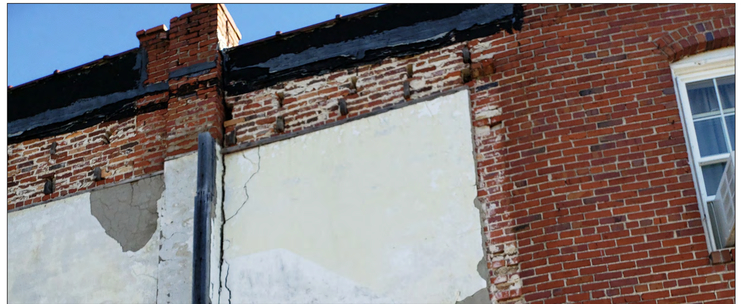
WEST FAÇADE CONDITION
