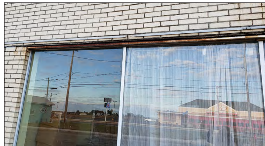
STORE FRONT LINTEL CONDITION
