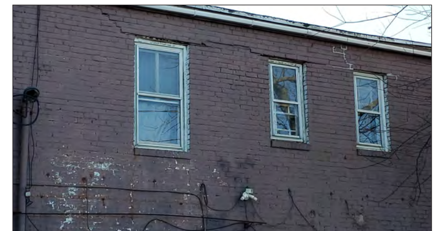
REAR FAÇADE CONDITION
