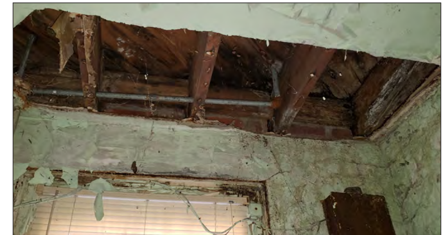
2ND FLOOR FRAMING LINTEL DAMAGE
