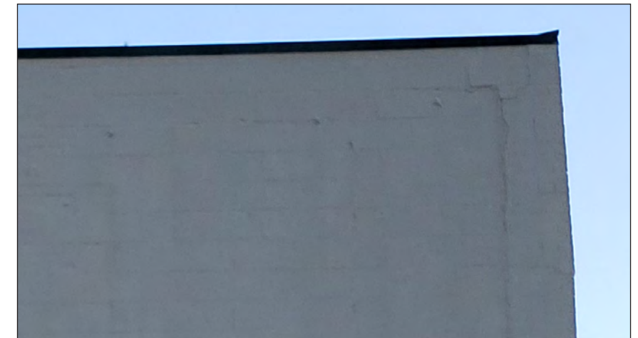
CRACKED/RACKING MASONRY
