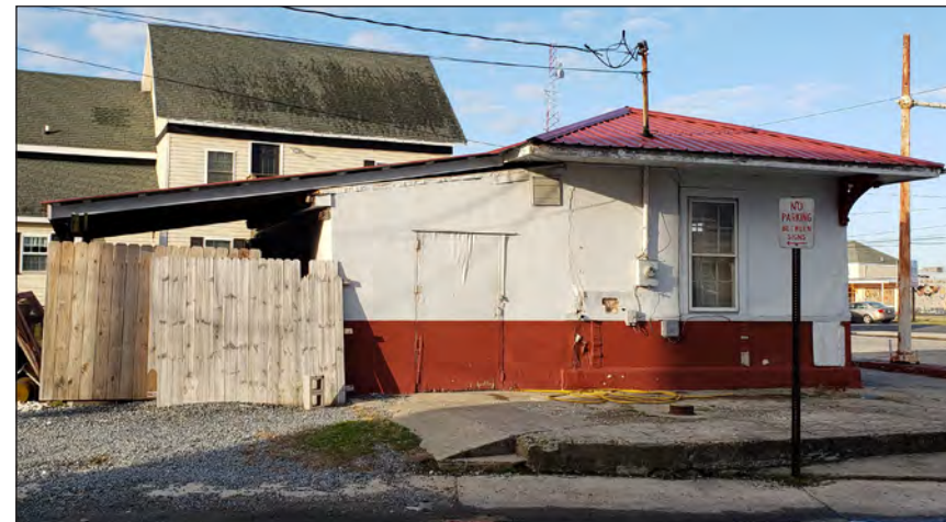
WEST FAÇADE CONDITION
