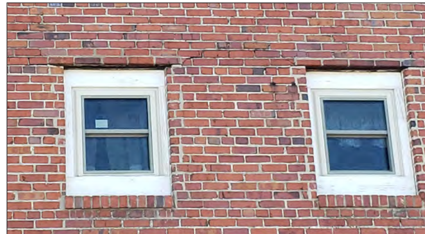
TYPICAL LINTEL CONDITION ON WEST FAÇADE
