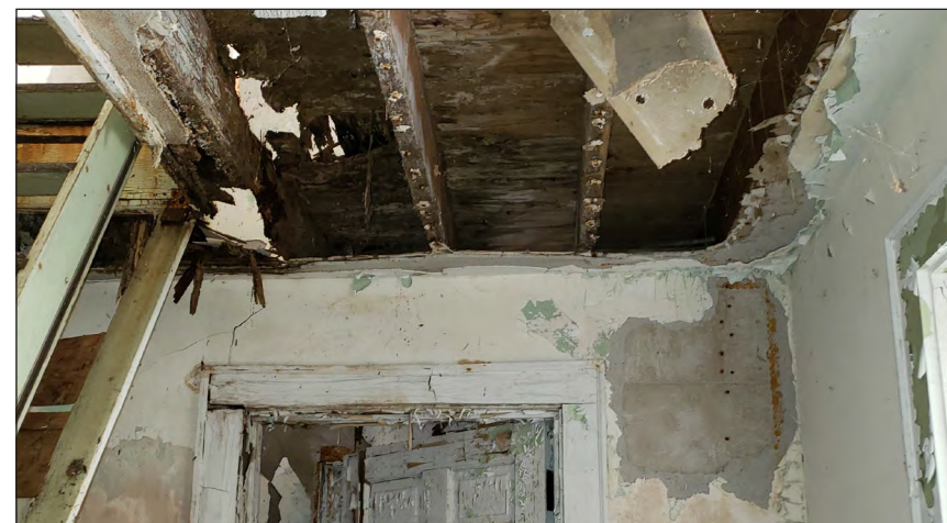
2ND FLOOR & STAIR DAMAGE
