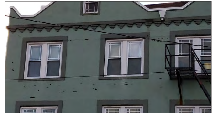
EAST FAÇADE CONDITION
