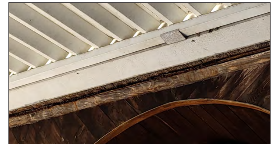
382 W. MAIN STREET STORE FRONT CONDITION
