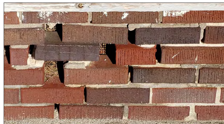
DISPLACED MASONRY UNITS
