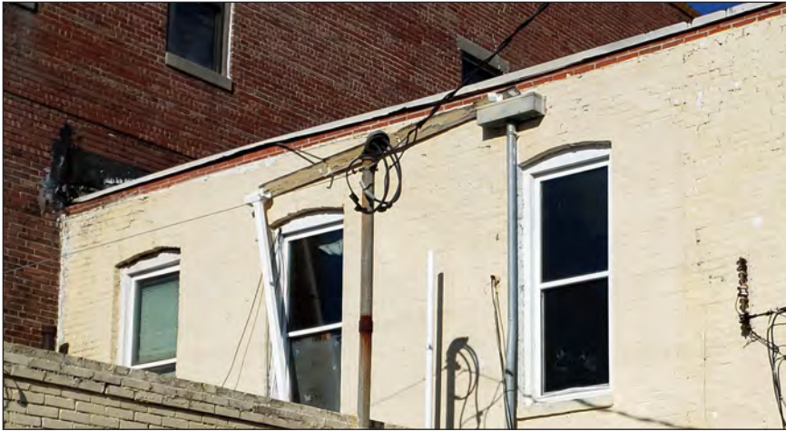
REAR FAÇADE CONDITION
