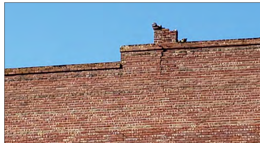
EAST FAÇADE CONDITION
