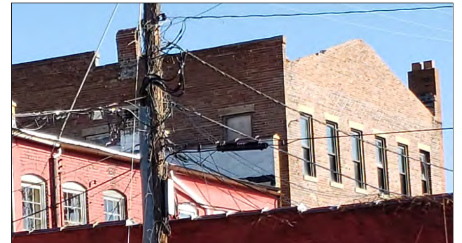
WEST FAÇADE CONDITION
