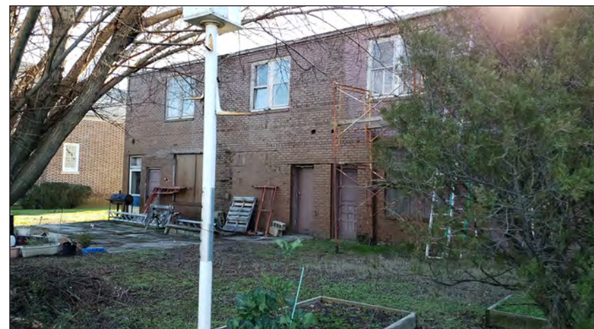
REAR FAÇADE CONDITION
