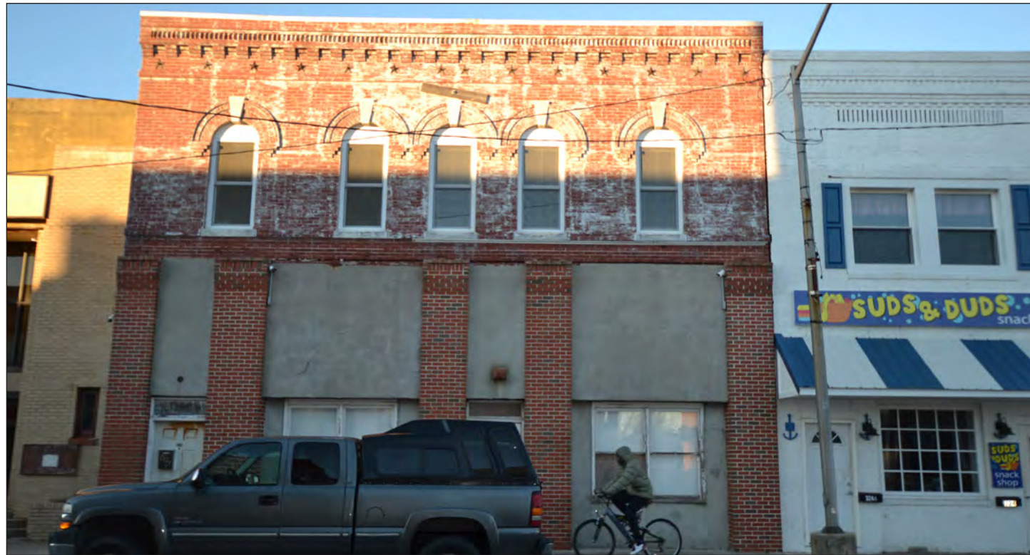
TYPICAL EXTERIOR CONDITION
