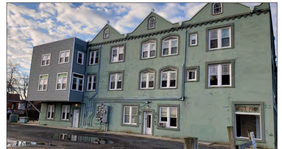
EAST FAÇADE CONDITION
