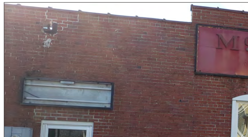
REAR OF BUILDING CONDITION
